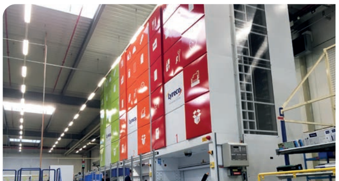
Fire protection system integration
